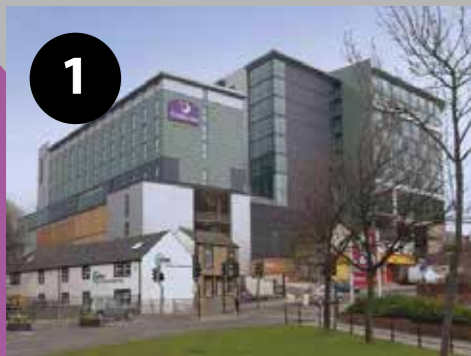
1 View of Premier Inn and Gateway Plaza from the Townend Roundabout.
