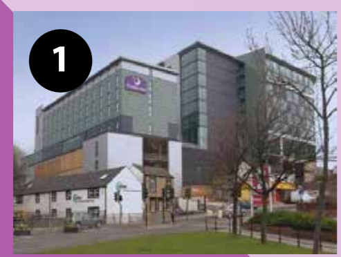
View of Premier Inn and Gateway Plaza from the Townend Roundabout.
